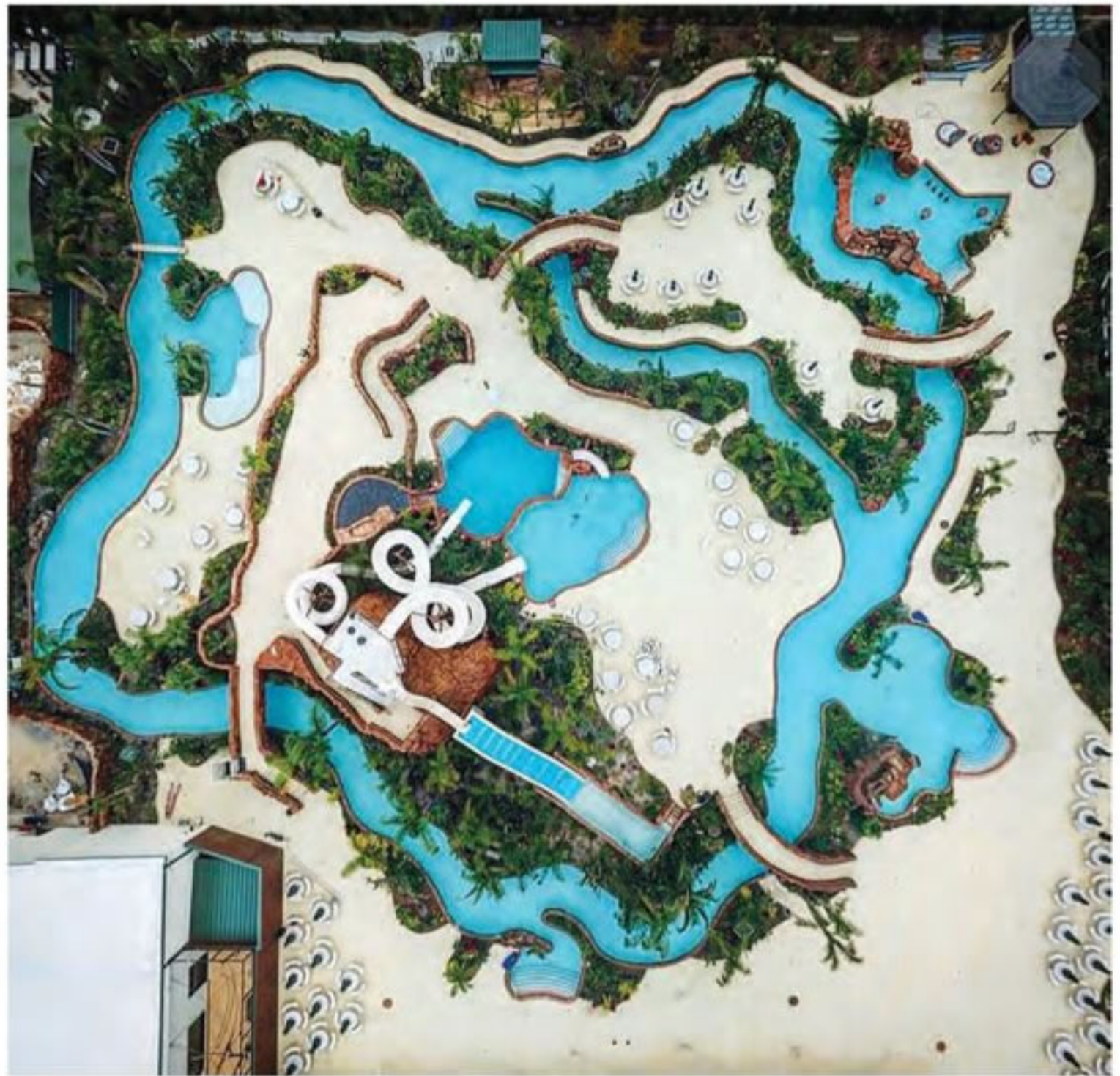
Houston's Club Westside, designed by Counsilman-Hunsaker & Associates and built by Progressive Commercial Aquatics, has Riverflow Pumps.
